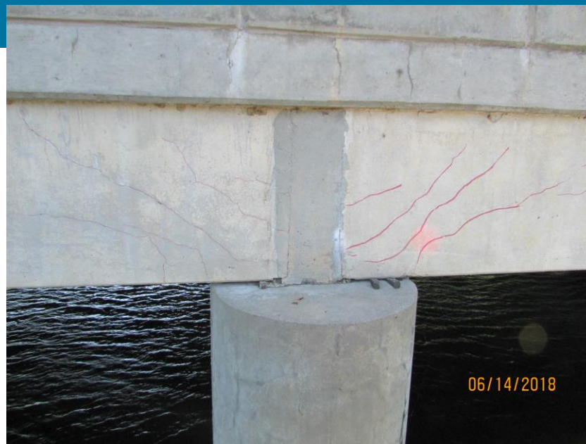
CRACKS IN FASCIA BEAMS AT PIER
