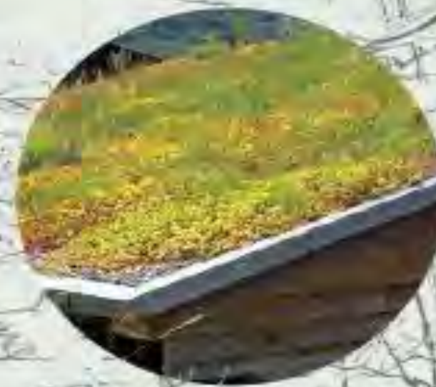
EXTENSIVE GREEN ROOF
