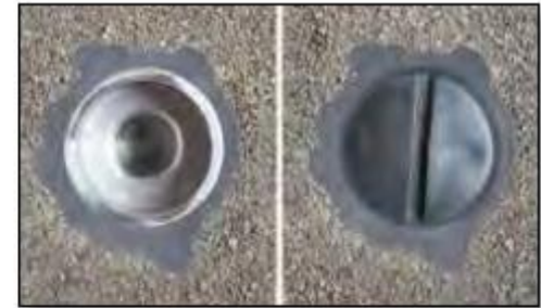
The anchor cup securely installed shown with and without plug cap
